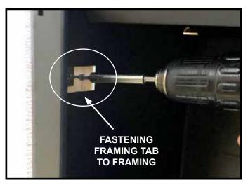
Figure 4.13 Fastening Framing Tab to Framing
